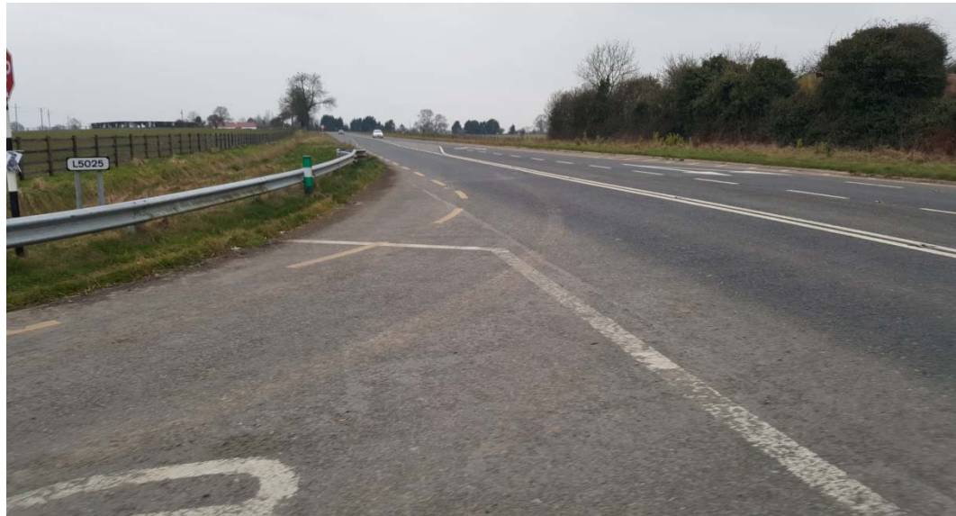
Plate 13.1.2 – Location 1 – R402 / L-5025 Derrymahon Junction, looking south west along R402
